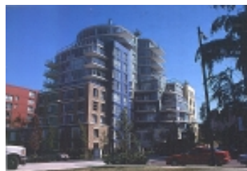
Apartments with ground floor active uses mixed with office space enhance on-street retail frontage and support live/work communities. (Vancouver, B.C.)
