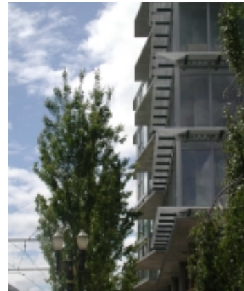
Cascadian condominiums Phase I nearing completion, 2001.
