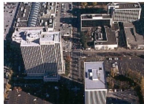
Parking lots are often vacant after hours because of insufficient District activities. Parking primarily serves employees and events at the OCC and Rose Quarter.
