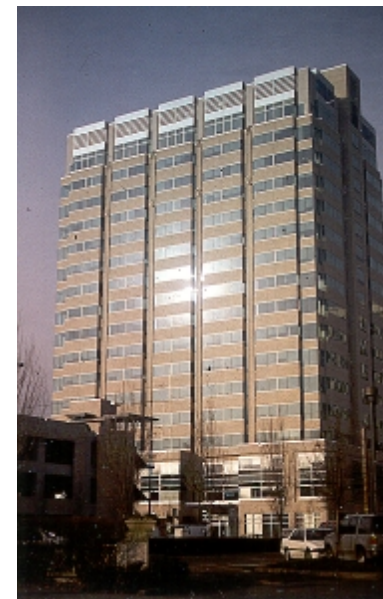
Liberty Centre office tower.
