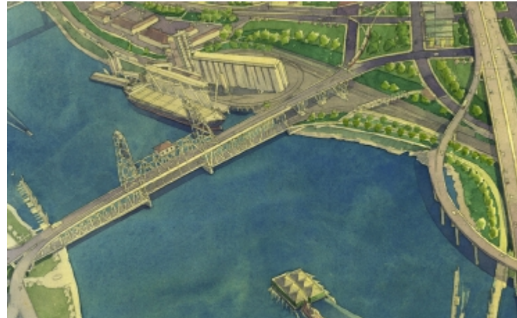
The Steel Bridge RiverWalk improvements on the lower deck provide convenient pedestrian and bicycle connections between the Lloyd District, Waterfront Park and the Eastbank Esplanade.
