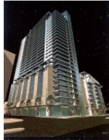
Cascadian condominiums at Northeast Grand and Holladay. The first phase, an 8-story block, began construction in Fall 2000.
